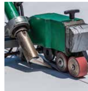
Heat Welding Seams
